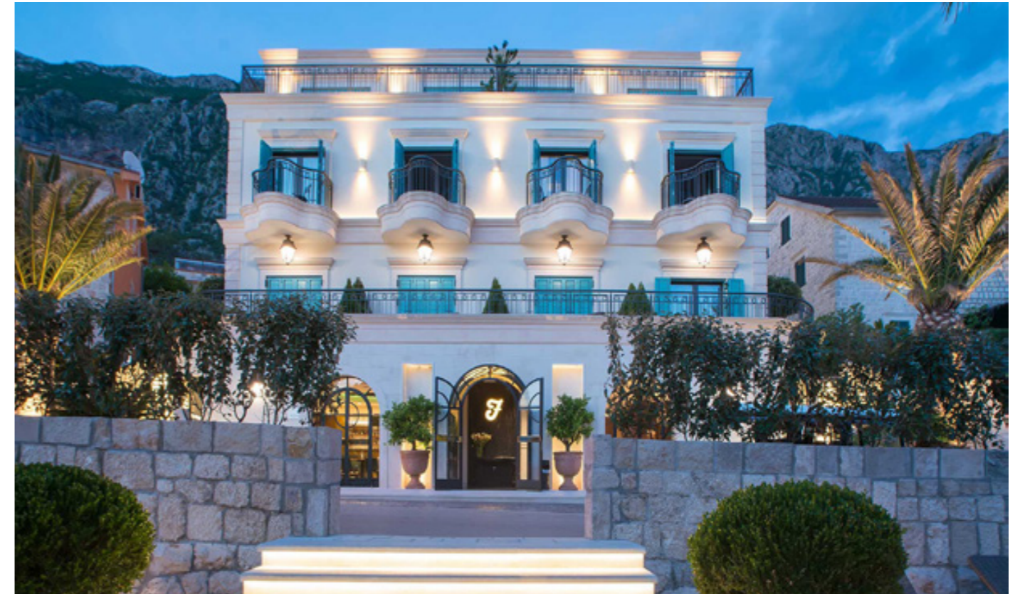
FORZA TERRA Boutique Hotel & Spa ***** Kotor, MNE
